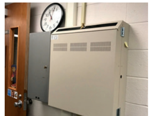
(Photos show the size of the equipment rack removed from Central Elementary that was replaced with the slim wall mount cabinet)
